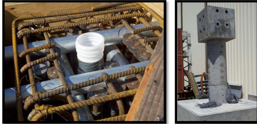
Figure 50. Construction of the upper portion of the column and the load stub.
