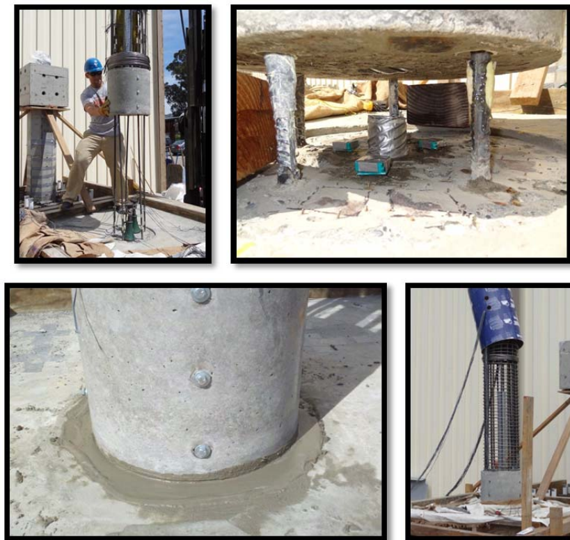
Figure 49. Installation of the precast HyFRC end portion.
