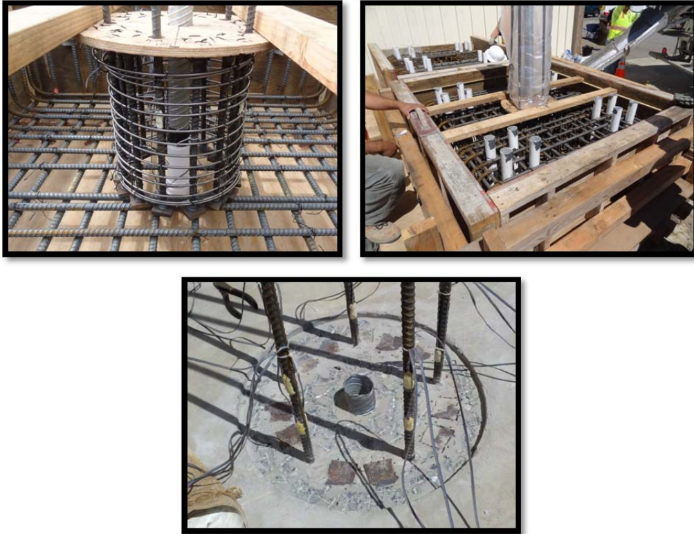
Figure 48. Construction of the footing.
