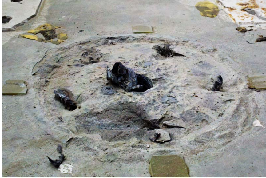
Figure 72. Grout pad after column demolition.
