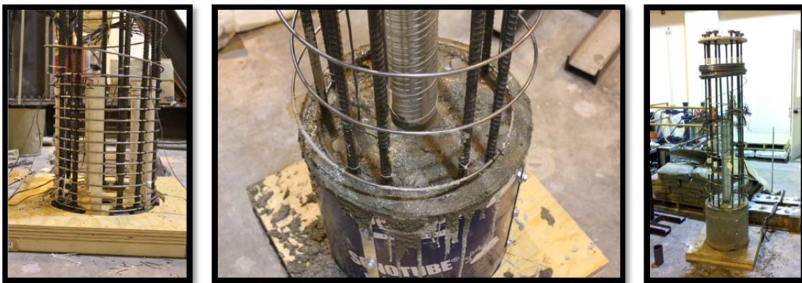
Figure 47. Construction of the precast HyFRC column section.
