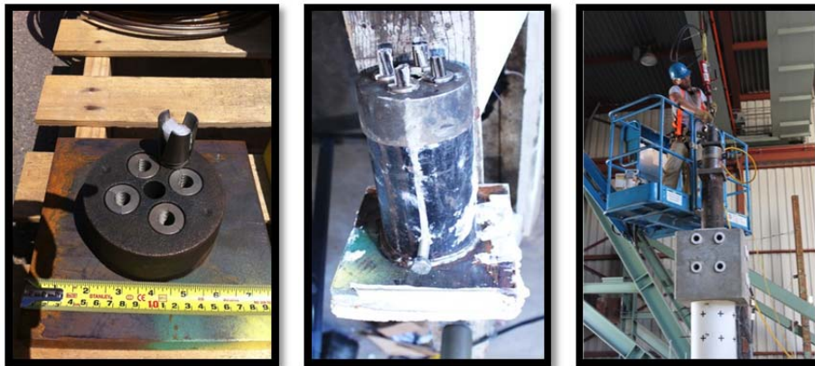
Figure 51. Strand anchorage and stressing.
